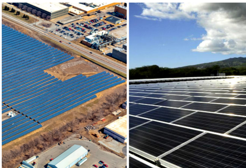
10.86-MW Maywood Solar Farm in Indianapolis (Left) and 5-MW Kalaeloa Renewable Energy Park in Hawaii, U.S.A. (Right)
