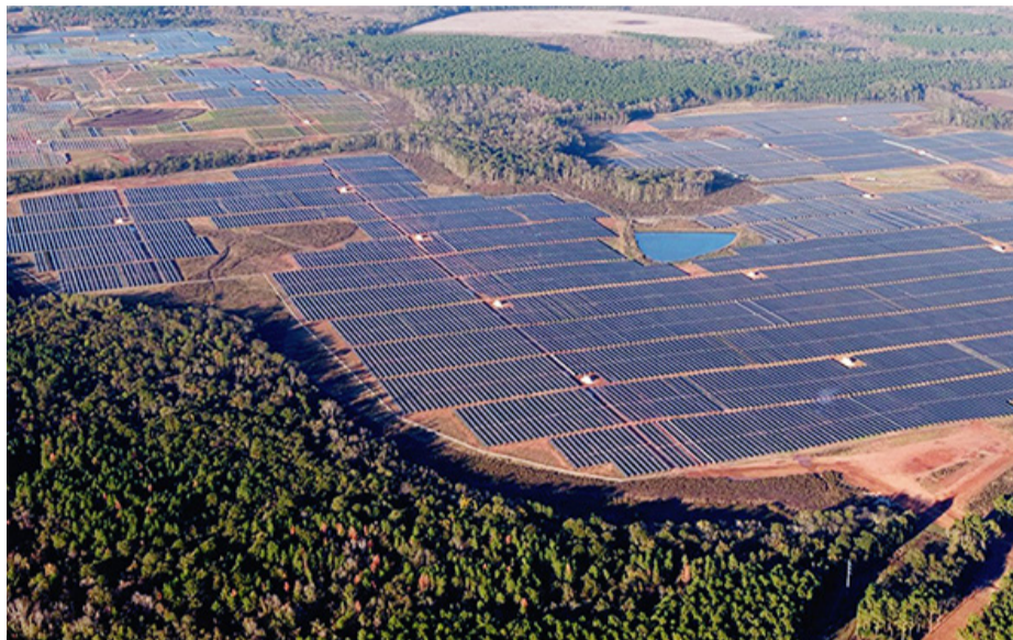
102.5-MW solar farm powering Facebook’s ninth data center in Georgia, U.S.A.
