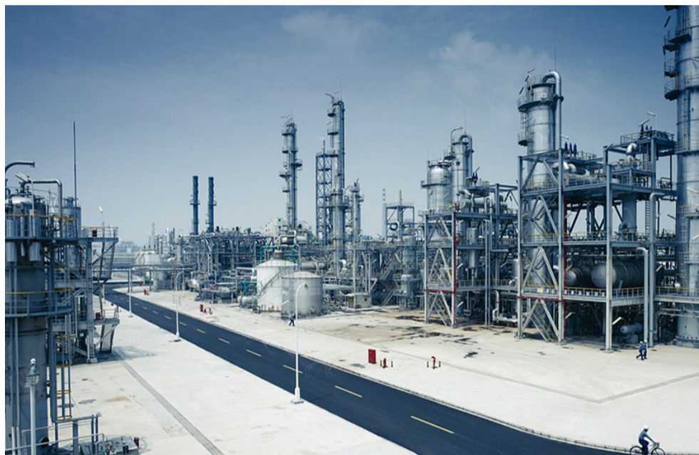
Hanwha Solutions' Chemical Division's plant in Ningbo, China
