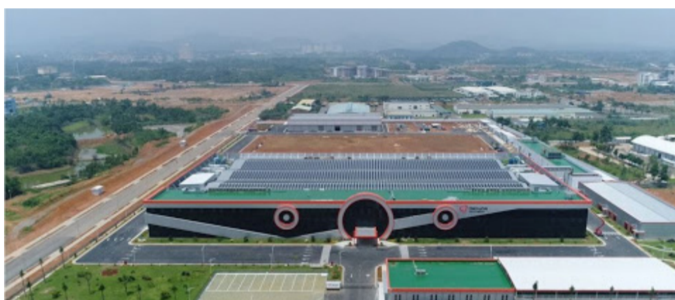
Hanwha Aero-Engines factory in Vietnam
